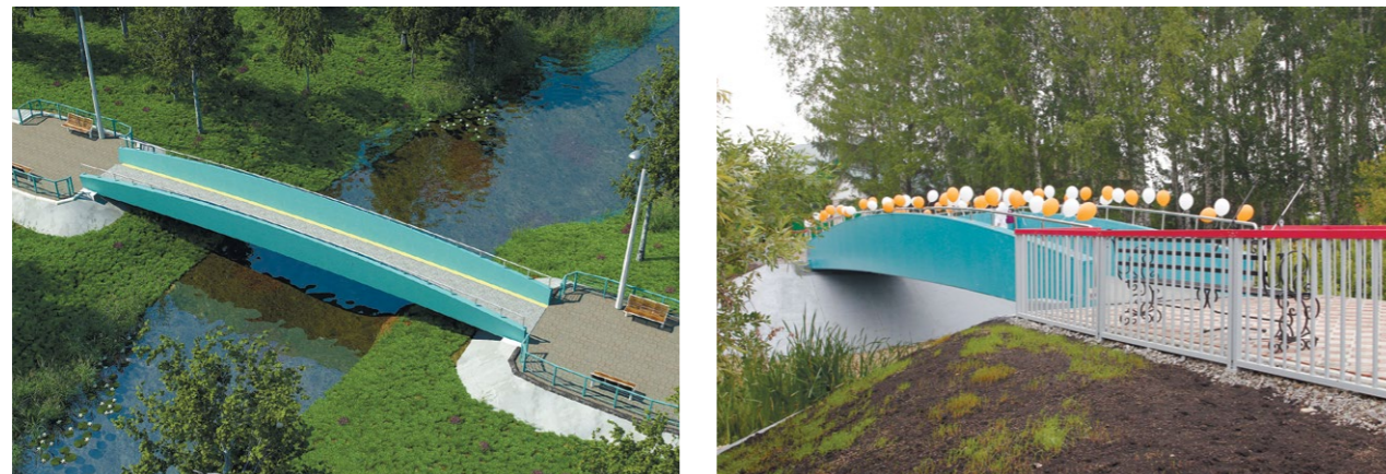
Pedestrian bridge over a river in Starobaltachevo village, Republic of Bashkortostan
