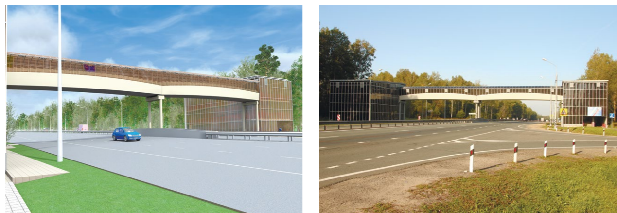
Pedestrian bridge, 250 km of M-1 Belarus highway
